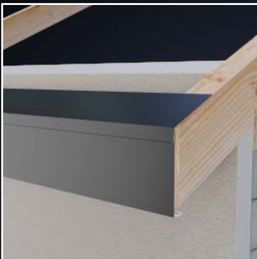
Installation of a gutter (condensate) belt.
