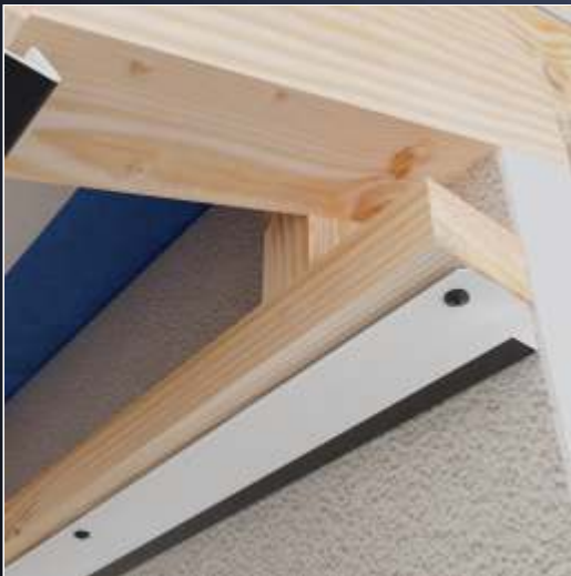
Installation of J-strip to the roof board. We recommend installation with staples for sheet metal.
