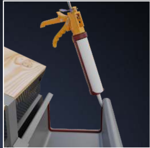
Sealing the gutter end with the use of an appropriate binder - application of binder onto the gutter.
