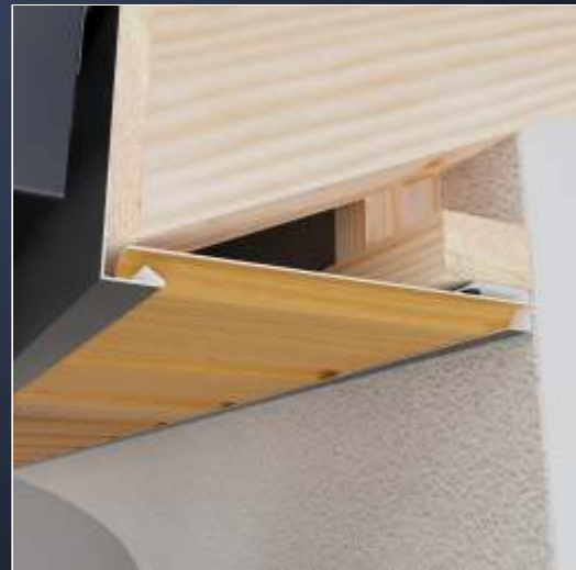
A soffit lining mounted on the flashings.
