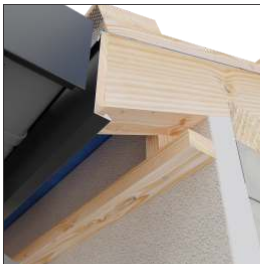
Installation of a rack for the mounting of the soffit lining.
