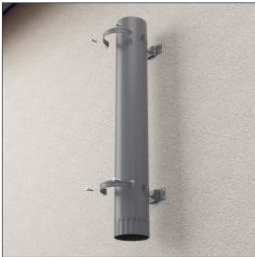
Installation of a drain pipe in clamps, connecting of a drain pipe with a coupling.
