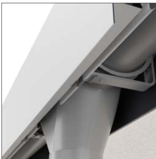
The cover plug is properly attached to the clips.
