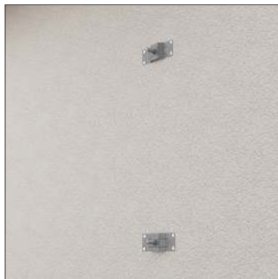
In the case of non-insulated buildings or buildings with walls, e.g. made of sandwich panels, clamp plates can be used, which are attached directly to the facade.
