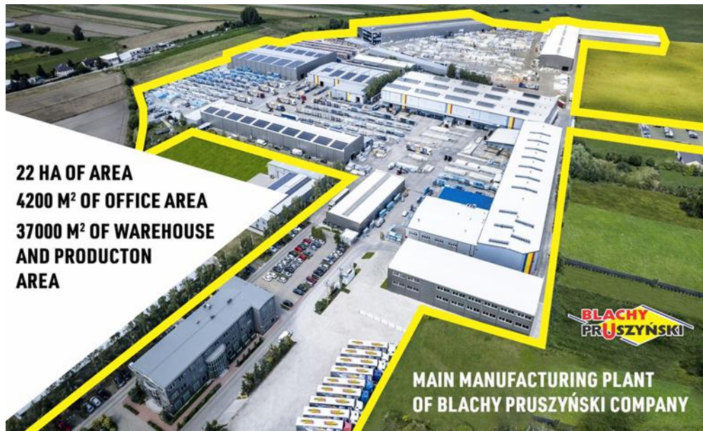
Figure 3.1: A view of the Pruszyński Sp. z o.o. production hall
